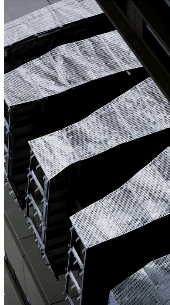
Above: CH2 has sustainable technologies integrated into every conceivable part of its 10 storeys.
