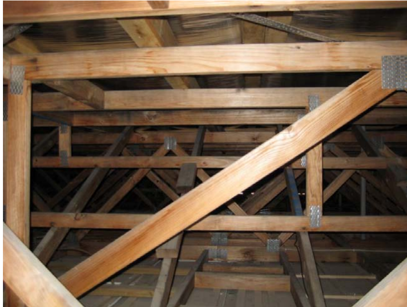
Roof truss system
